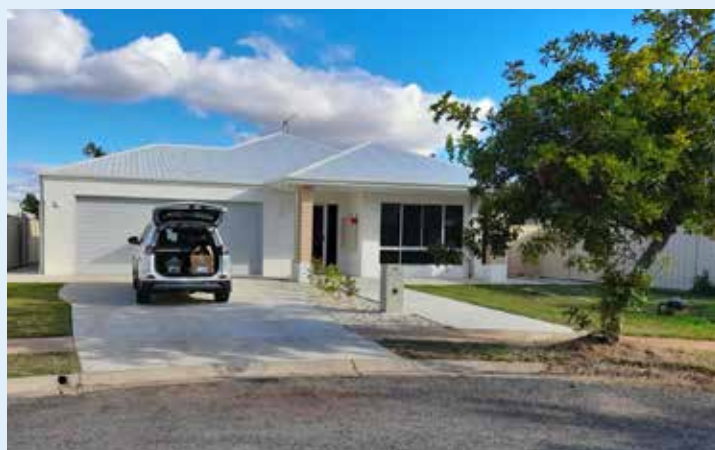
The house completed.
